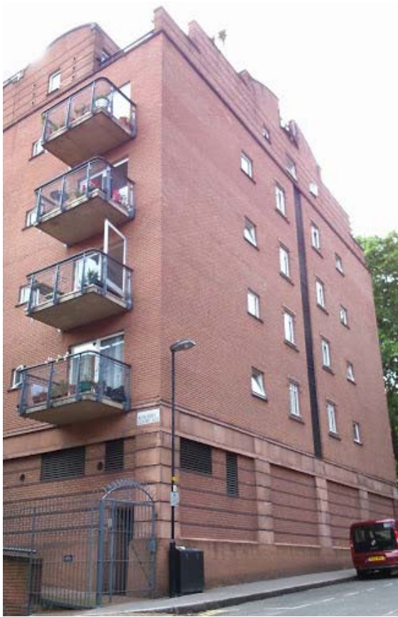
Rosebery Court, Coldbath Square
