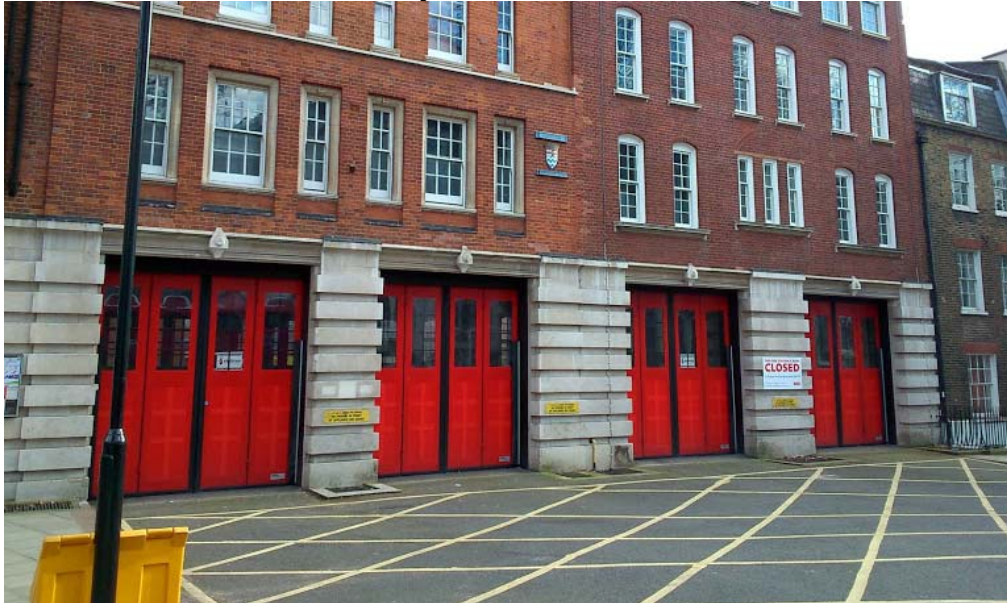
Fire Station Forecourt – Rosebery Avenue
