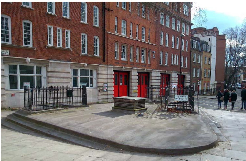
Underground former public toilets, Rosebery Avenue
