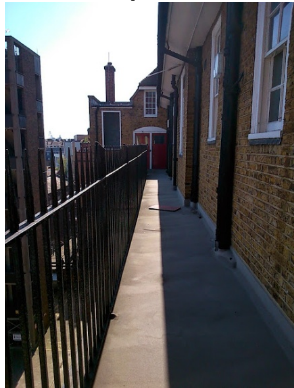
Iron railed rear landings
