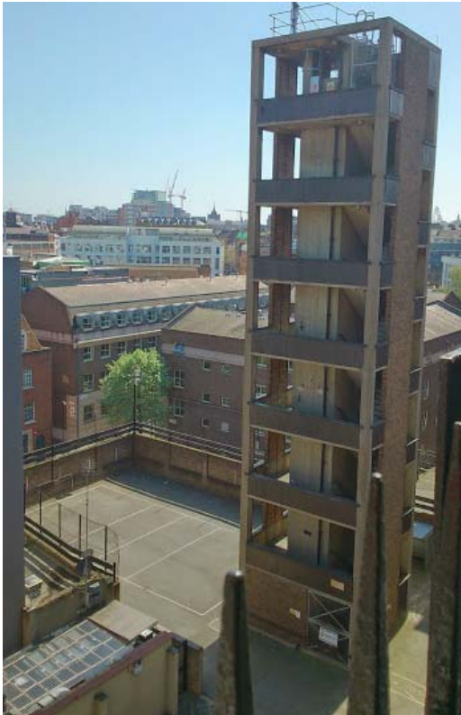
Modern drill tower
