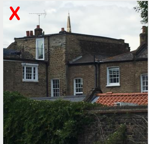
Figure 22 The roof extensions in the top image have been designed in a style appropriate to the host buildings and to maintain the prevailing roofline. In contrast, the roof extension in the bottom image projects significantly above the prevailing roofline and its size and treatment does not respect the scale and form of the host building or the rhythm of the wider terrace.
