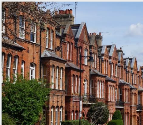
Red brick terrace on Baalbec Road, typical of the later Victorian period
