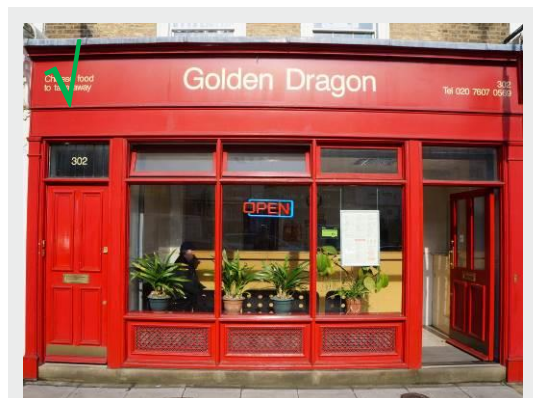
Figure 35 When ventilation grilles are proposed to a traditional shopfront they should be sensitively integrated into the stallriser.
