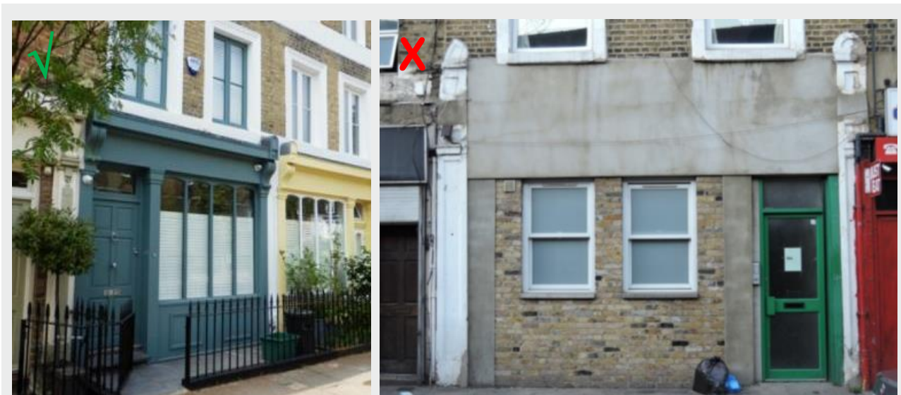
Figure 38 The conversion on the left has retained the external features of the original shopfront, using internal blinds to achieve privacy, to successfully introduce a residential use without compromising the character of the immediate surroundings. In contrast, the conversion on the right has not responded to the character of the building or the immediate surroundings and has a negative impact on the area.
